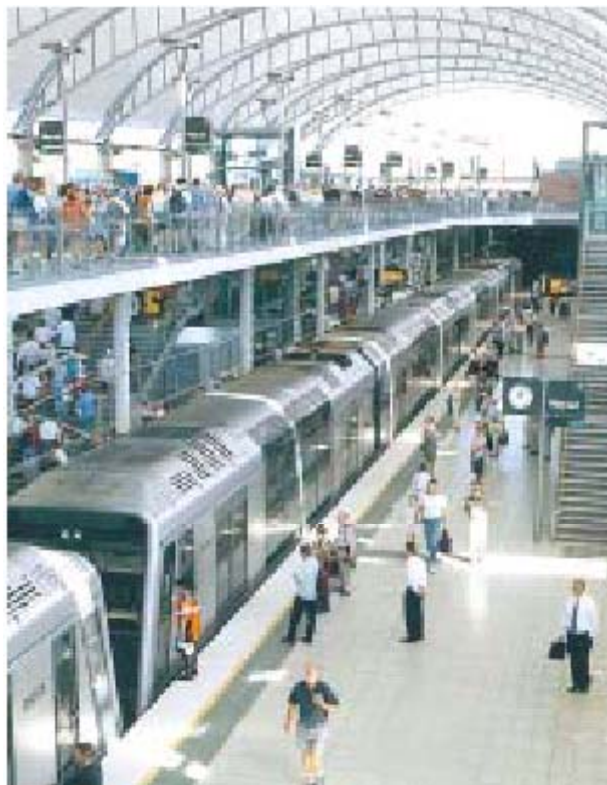
Rys. 12.6 - Olympic Park Station, Sydney
